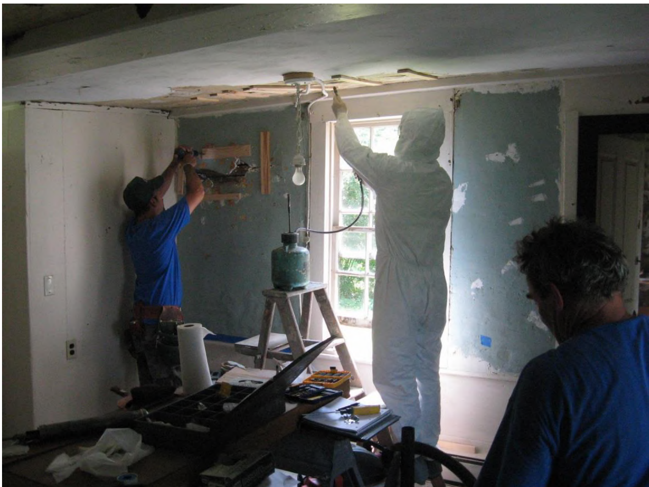
Fig. 14. Plaster conservation and repair in kitchen of Stekionis tenant farmhouse, Spencer-Peirce-Little Farm, 1690, Newbury, Massachusetts. ©Historic New England
