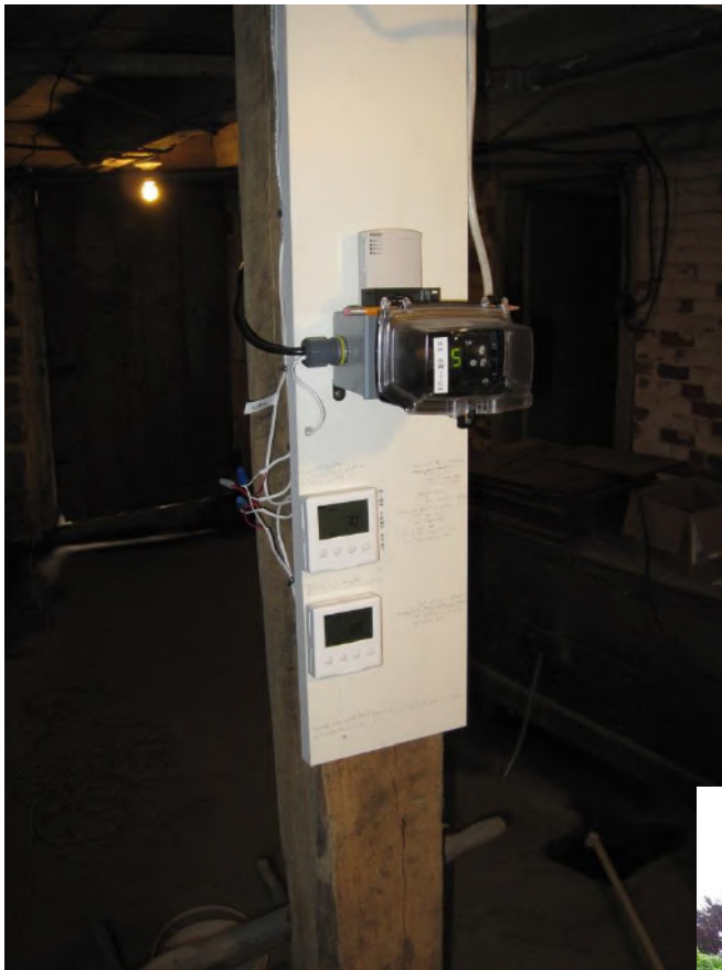
Fig. 12. Installation of a simplified environmental control system includes a thermostat and a humidistat. © Historic New England
