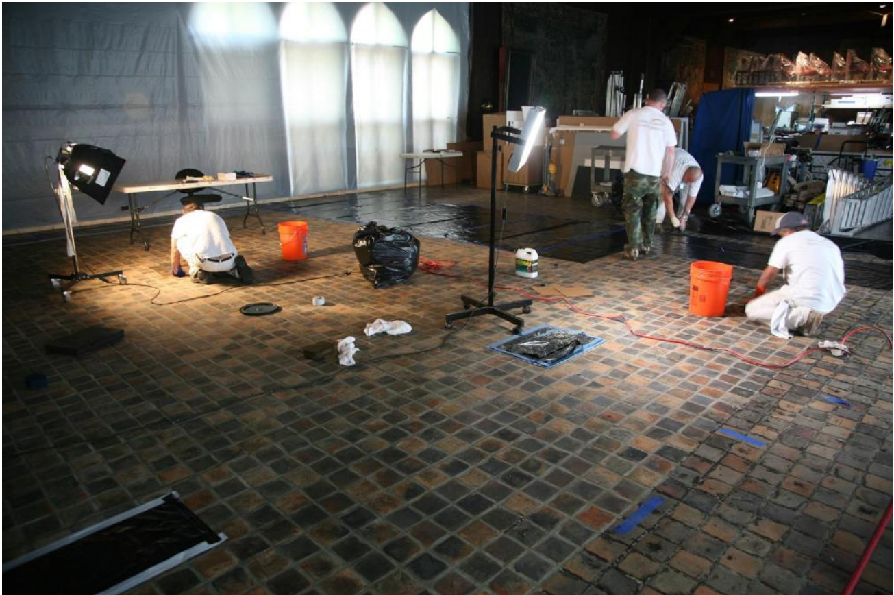
Fig. 7. Contractors removing old coatings from floor tiles.
