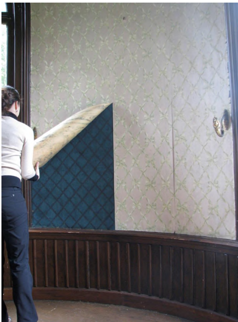
Fig. 6. Tower Room: wall with original 1860s wallpaper, and later 1950s wallpaper. ©E. Geldhof/R. Keppler
