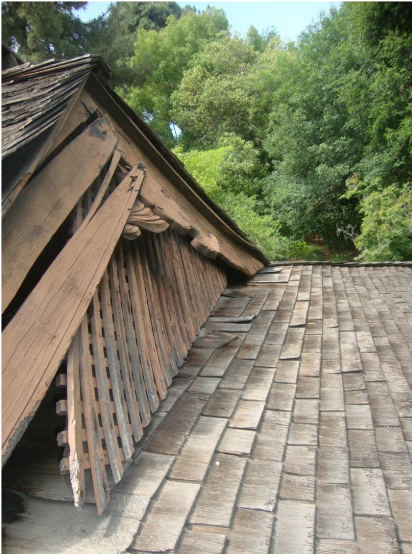
Fig. 3. Deterioration at the roof gable, ca. 2010. Courtesy of The Huntington Library, San Marino, California
