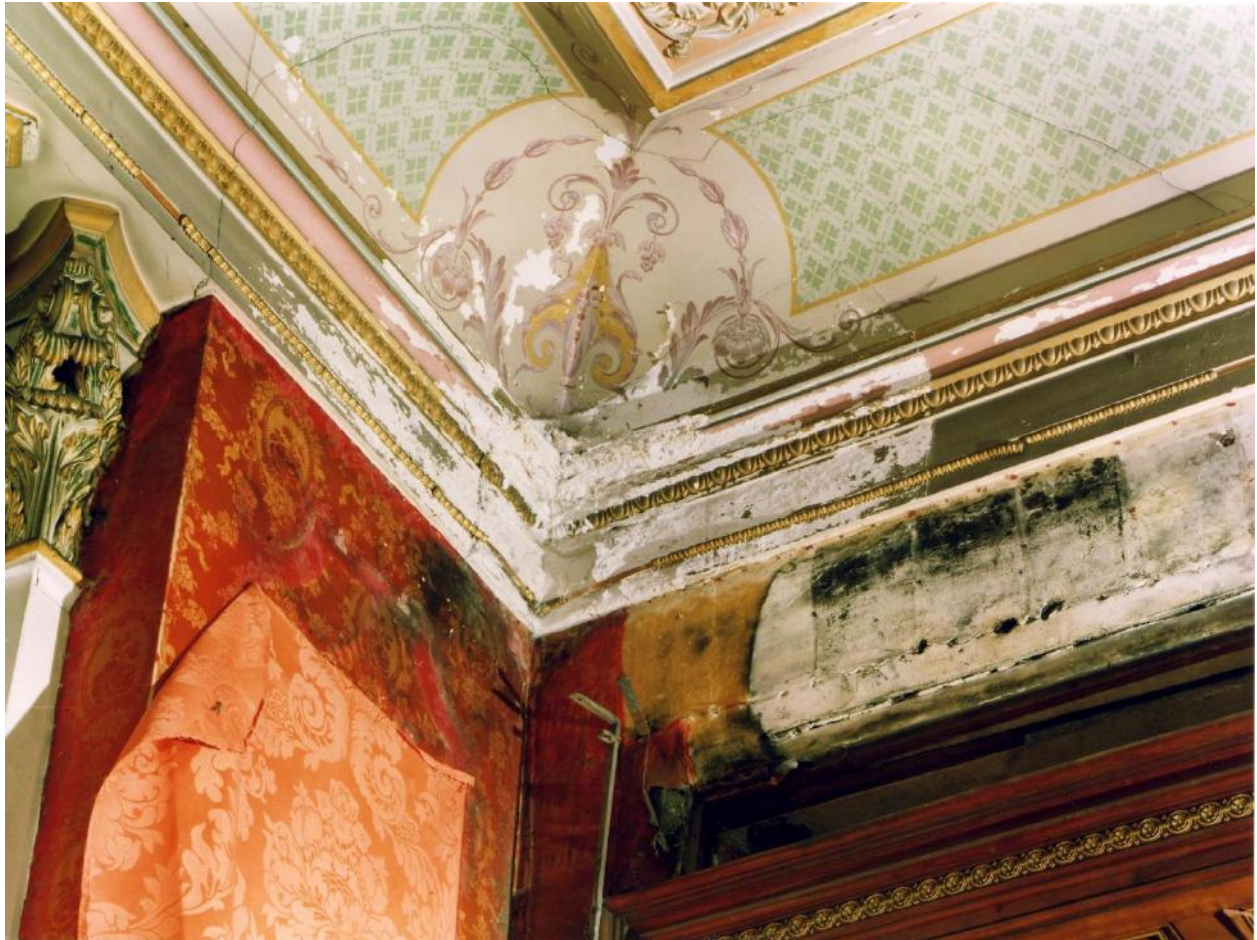
Fig. 6. Damage caused by water ingress. © English Heritage.
