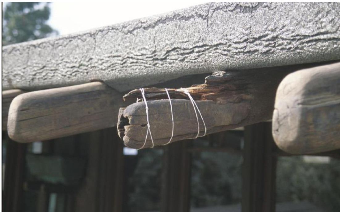
Fig. 2. Rafter tails before restoration. Courtesy Historic Resources Group
