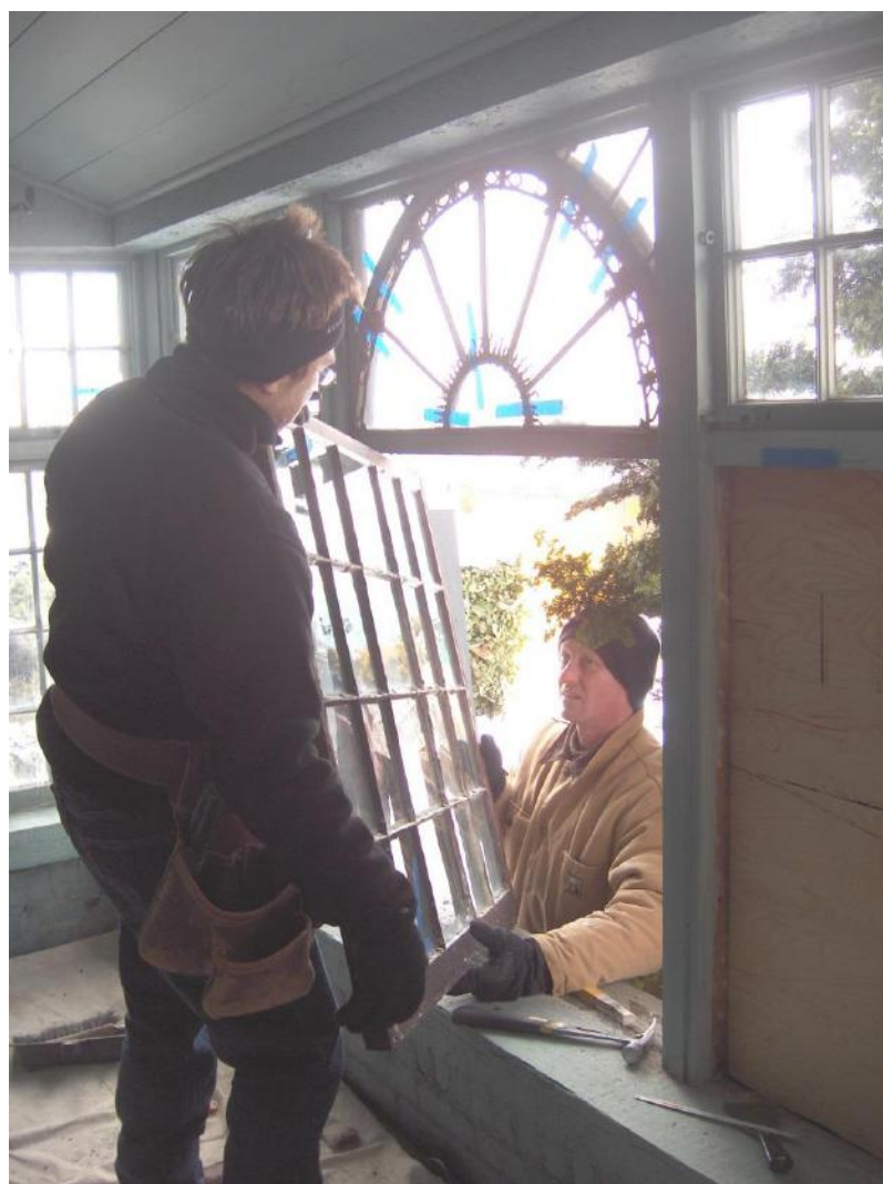
Fig. 10. Windows being removed for conservation work at Beauport. ©Historic New England
