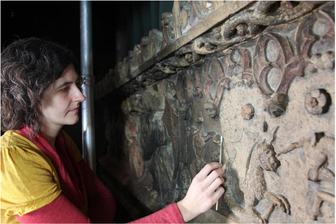
Fig. 6. Surface cleaning the fireplace.
