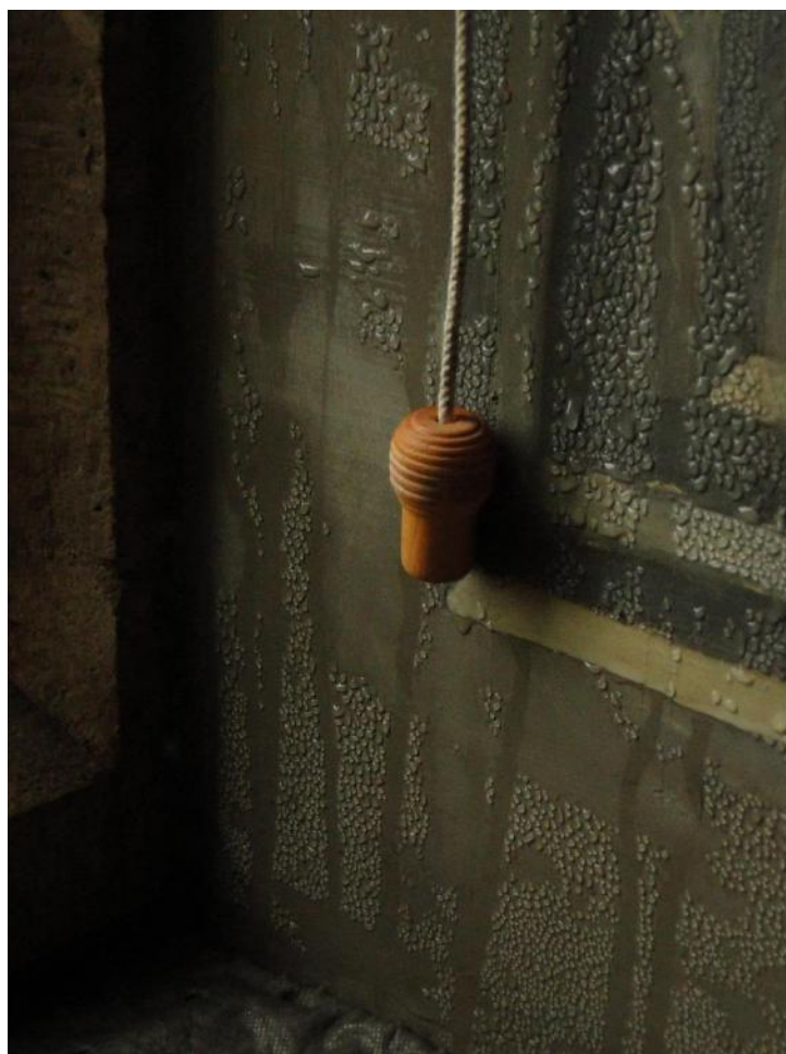
Fig. 3. Condensation on historic wall paintings, Knole. ©Emily Watts
