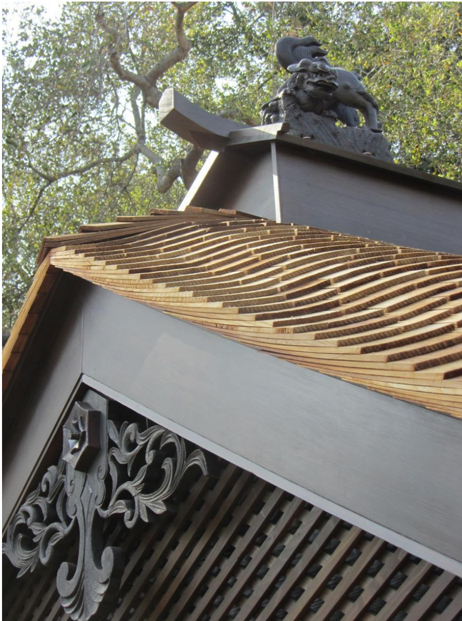
Fig. 7. Restored roof, gable vent, carved wood medallion, ridge box, and roof finial, 2012. ©Griswold Conservation Associates, LLC
