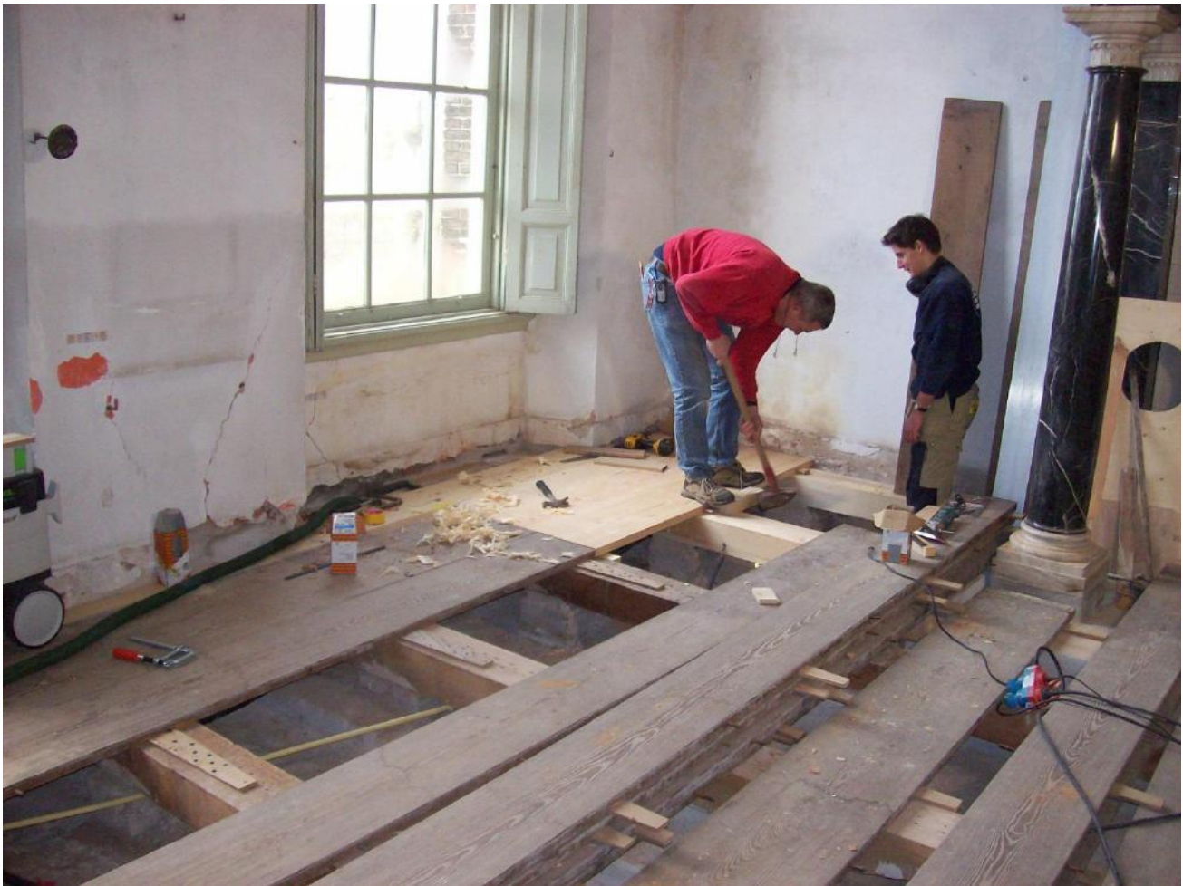
Fig. 5. Grote Zaal, drawing-room, original floor planks are re-positioned with wedges (2007).
