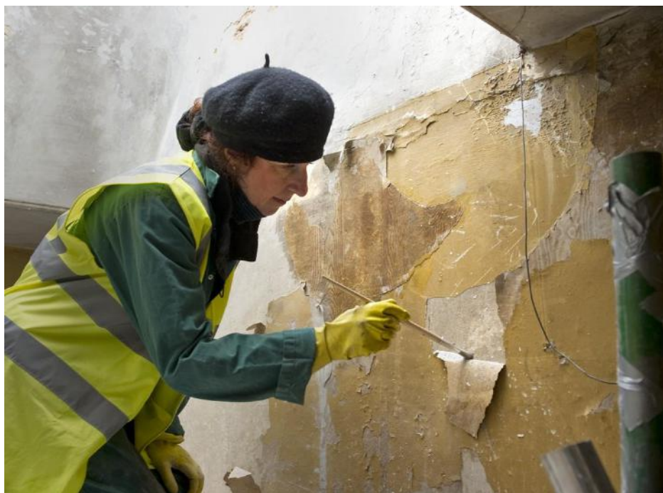
Fig. 6. Consolidation of interior surfaces. © English Heritage
