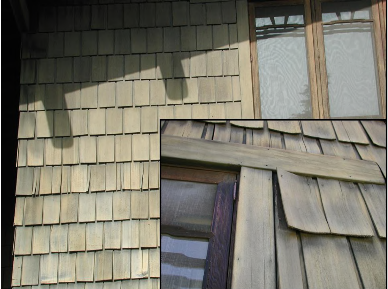
Fig. 5. Warped shakes before restoration. Courtesy Historic Resources Group
