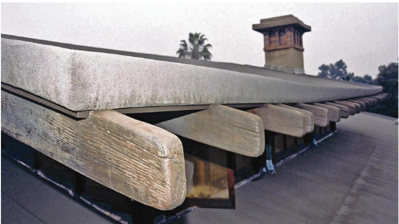
Fig. 3. Rafter tails after restoration. Courtesy Historic Resources Group
