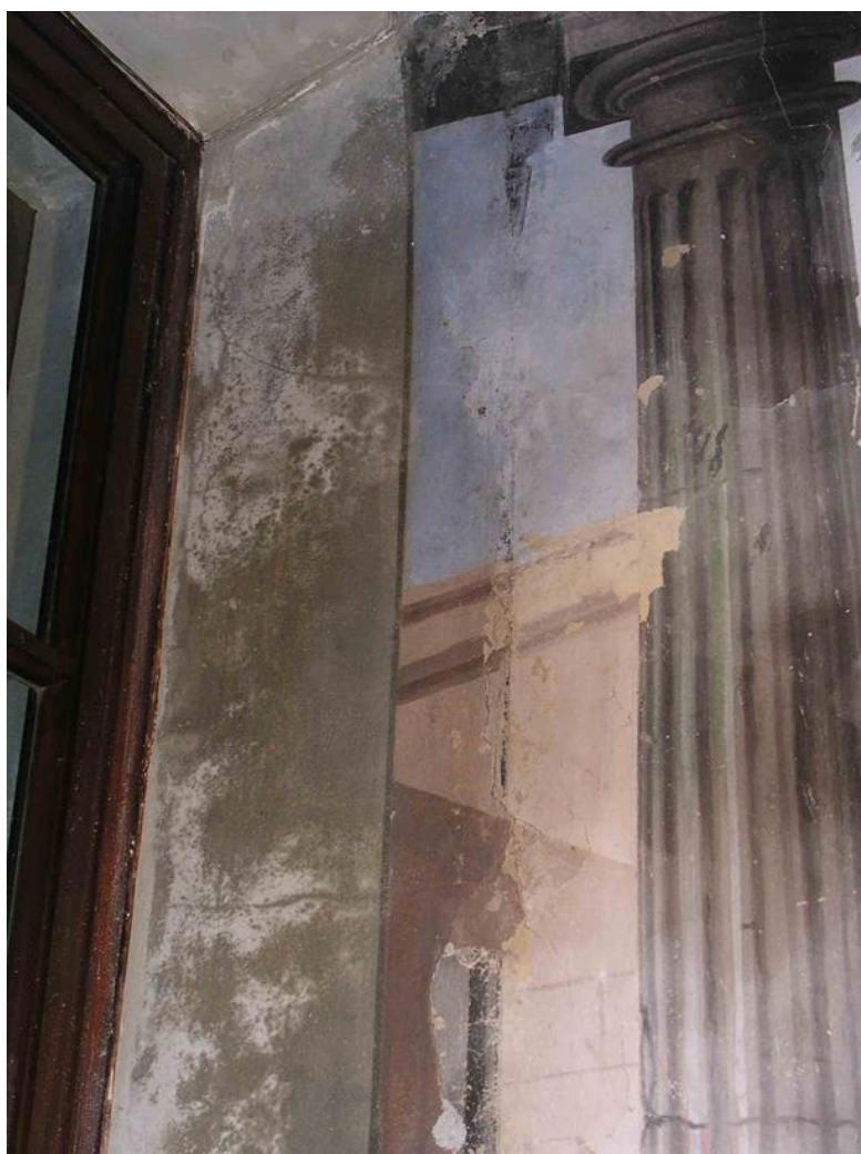
Fig. 12. Detail of deterioration around window. © New York University, Acton Collection, Villa La Pietra, Florence
