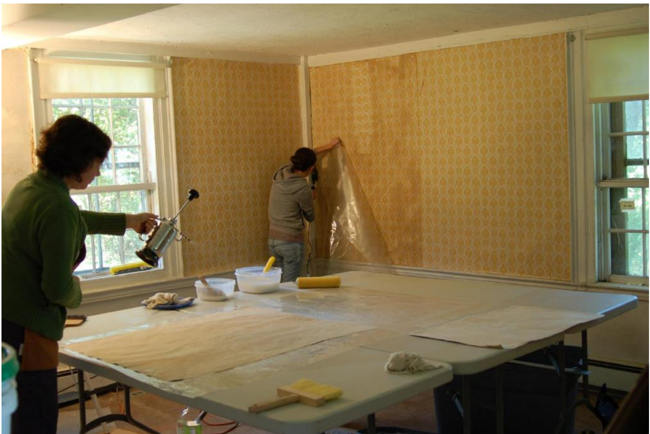
Fig. 15. Installation of conserved wallpaper in parlor of Stekionis tenant farmhouse, Spencer-Peirce-Little Farm, 1690, Newbury, Massachusetts . ©Historic New England
